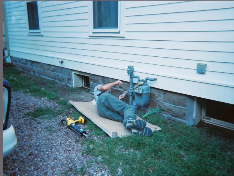
Battery caulking gun to apply final material
