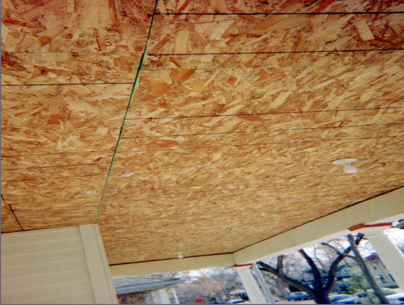
OSB in place – ready for primer & bead boards
