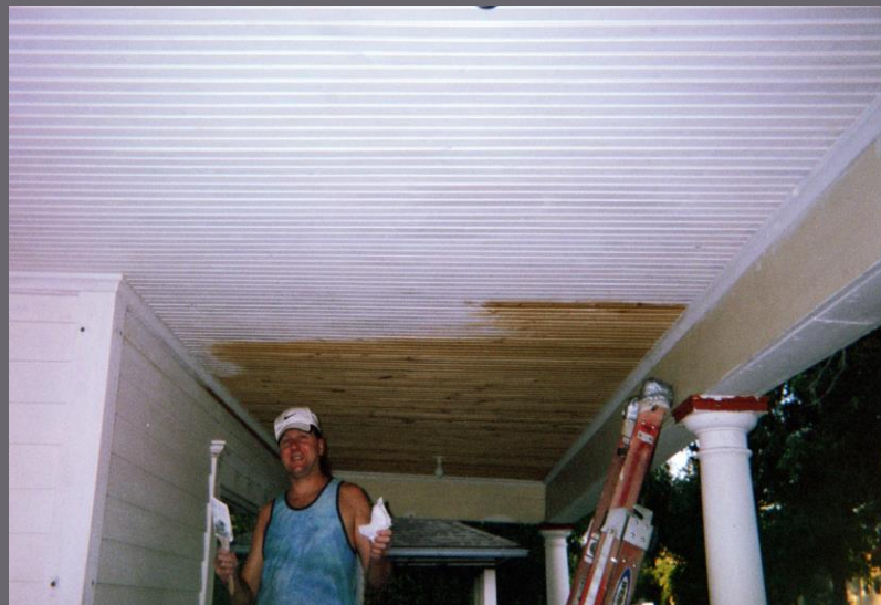
Tongue & groove knotty pine bead boards in place – ready for primer & paint
