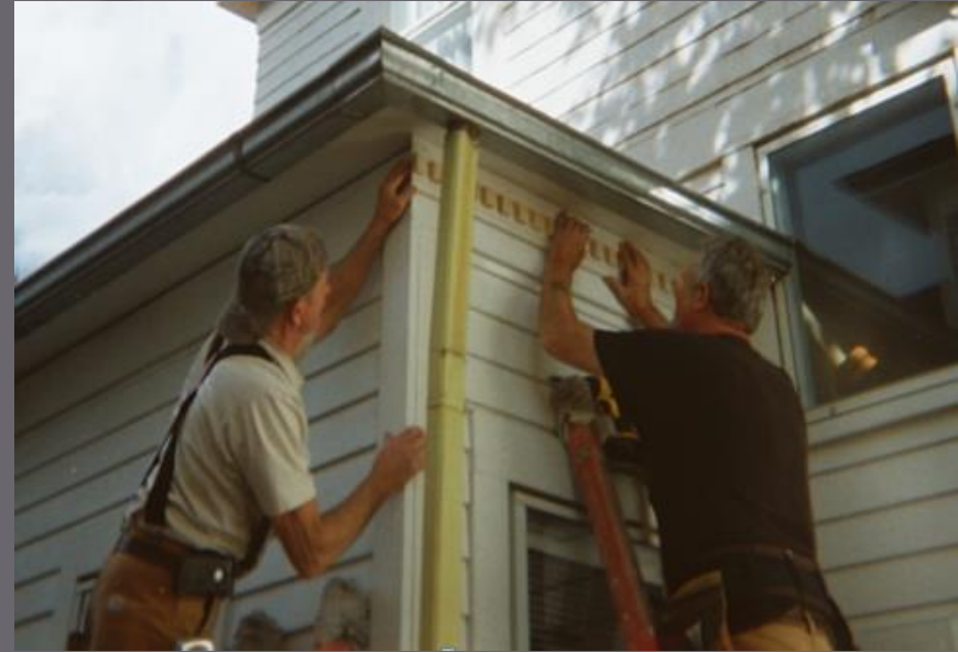
Installing dentil molding
