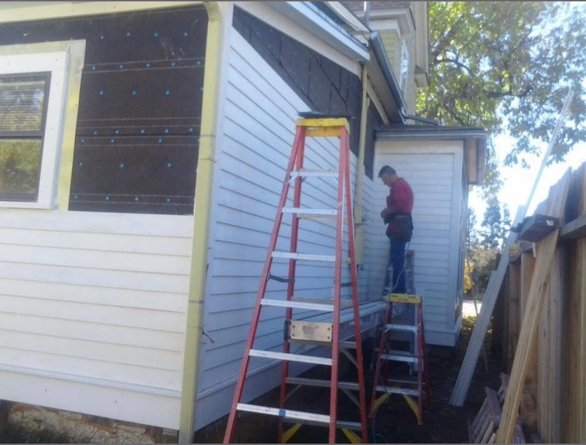
New clapboard are being installed
