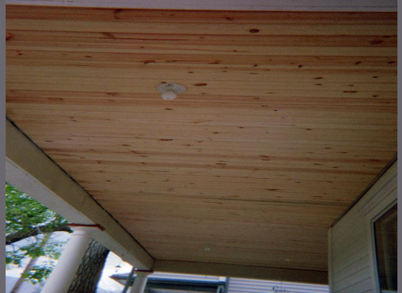
Tongue & groove knotty pine bead boards in place – ready for primer & paint
