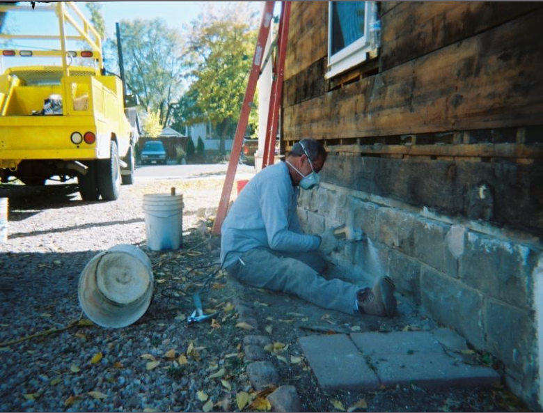
Grinding old mortar out
