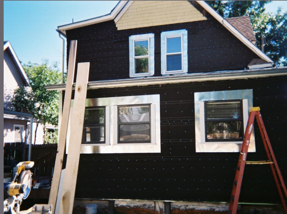
Tar paper in place and all windows and doors outfitted with tin flashing
