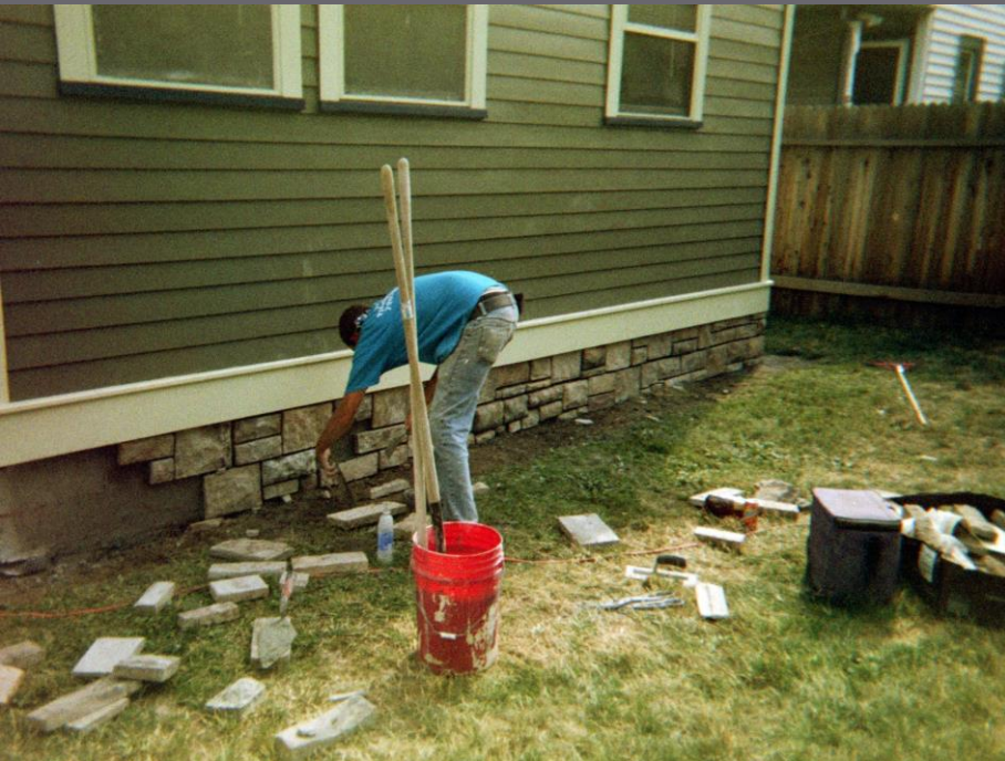
Building the new foundation wall with 'Cut Stone' to differentiate from the 1900 foundation
