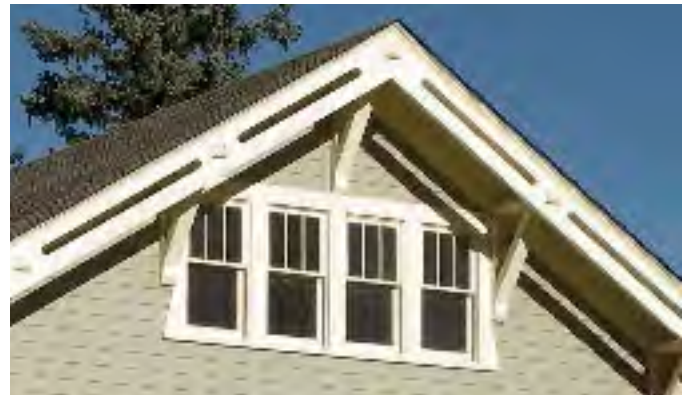
Grouped bungalow windows with triple pane upper sash.
