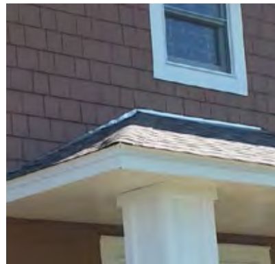
Flashing behind siding
