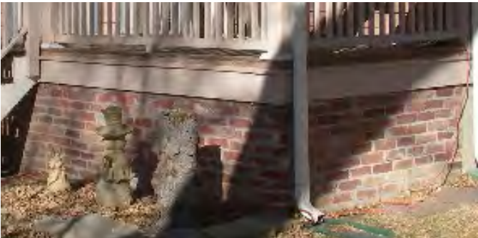
RECOMMEND the salvage and re-use of masonry as a veneer over new foundations. Maintain historic raised foundation relationship above ground.
