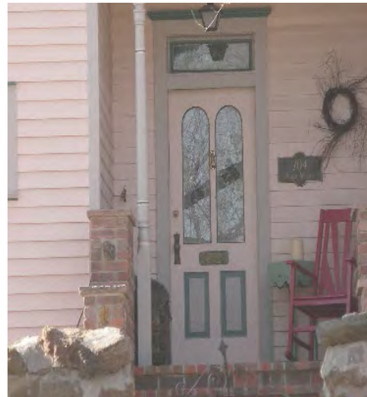
Preserved historic front door with arched top lites. Window above door is a transom lite.
