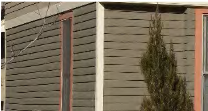
Exterior wall repaired by partial replacement of damaged bevelled cedar siding to match existing siding that has been retained and repaired.
