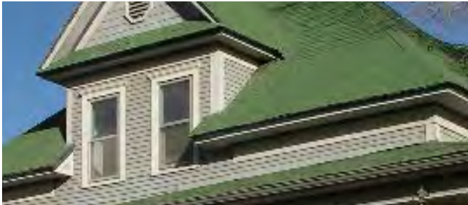
Example of well-maintained siding and trim. Trim occurs at wall corners, intersections of roof overhangs, around vents and around windows.
