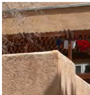
New colored stucco exterior wall finish.
