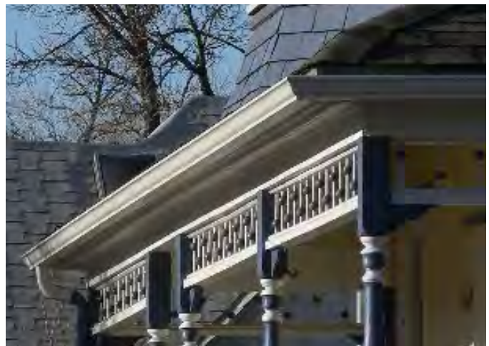
Example of gutters in good condition and connected to downspout to convey water away from building.
