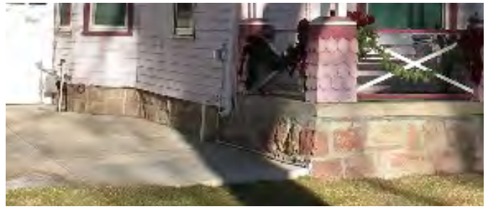
New replacement foundation that uses salvaged foundation stone as a veneer over new poured concrete foundation walls. Height of new foundation preserves the original podium relationship of height of floor above surrounding ground.
