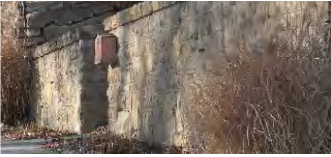
RECOMMEND using correct mortar repairs to match joint softness, joint size, and mortar colors.
